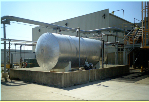
Steel Tank Containing Regulated Substance
