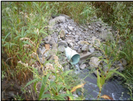
Lift pumps transfer runoff to detention pond
