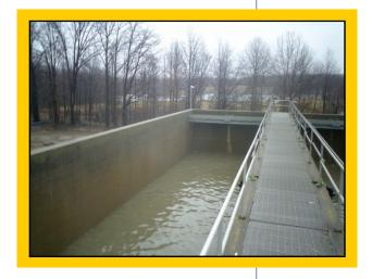
Our client, a publicly-owned treatment works in Lorain County, Ohio, was experiencing isolated events where the incoming flow exceeded the peak design flow for the treatment equipment. These high flow events caused overflows of the equalization tanks, which in turn caused soil erosion and property damage.
